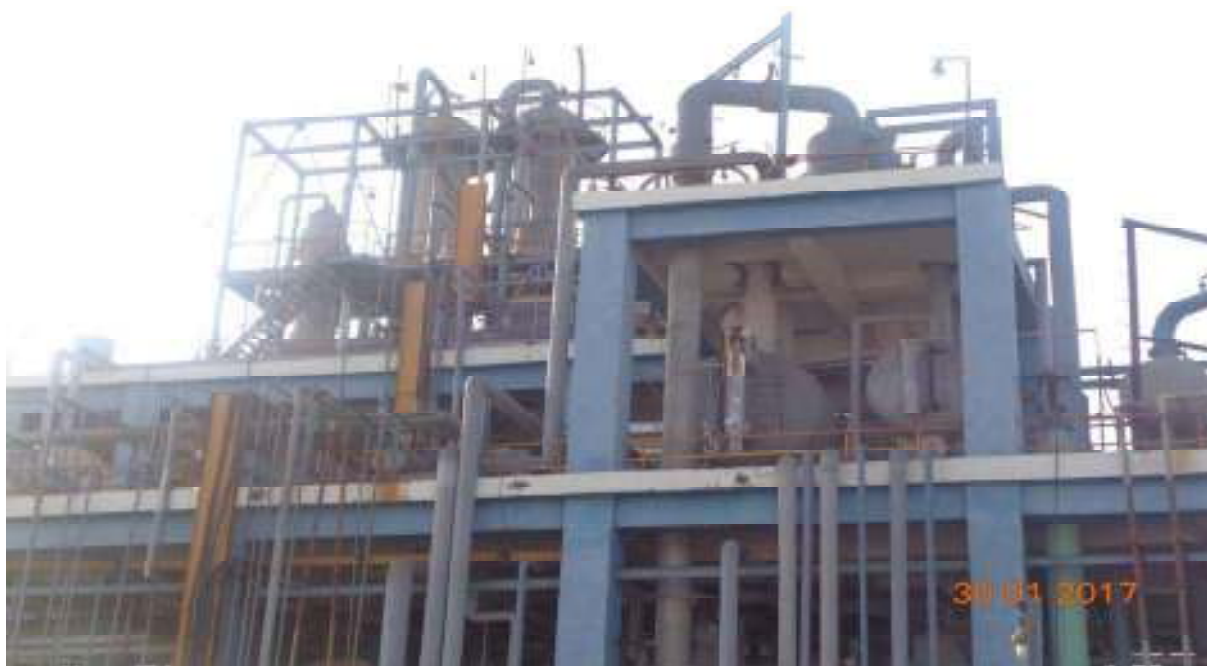
Scrubbing System for HCl generated from Chloromethane
