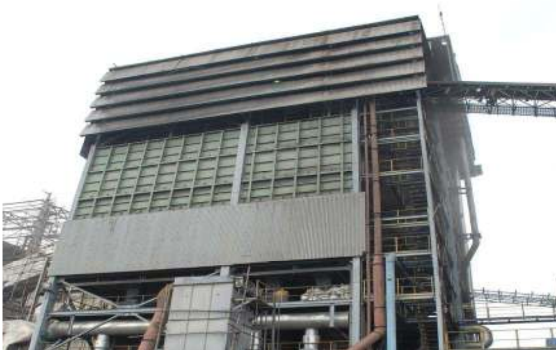
Fig 10.2 Photographs of Bag Filter of Dust extraction system
