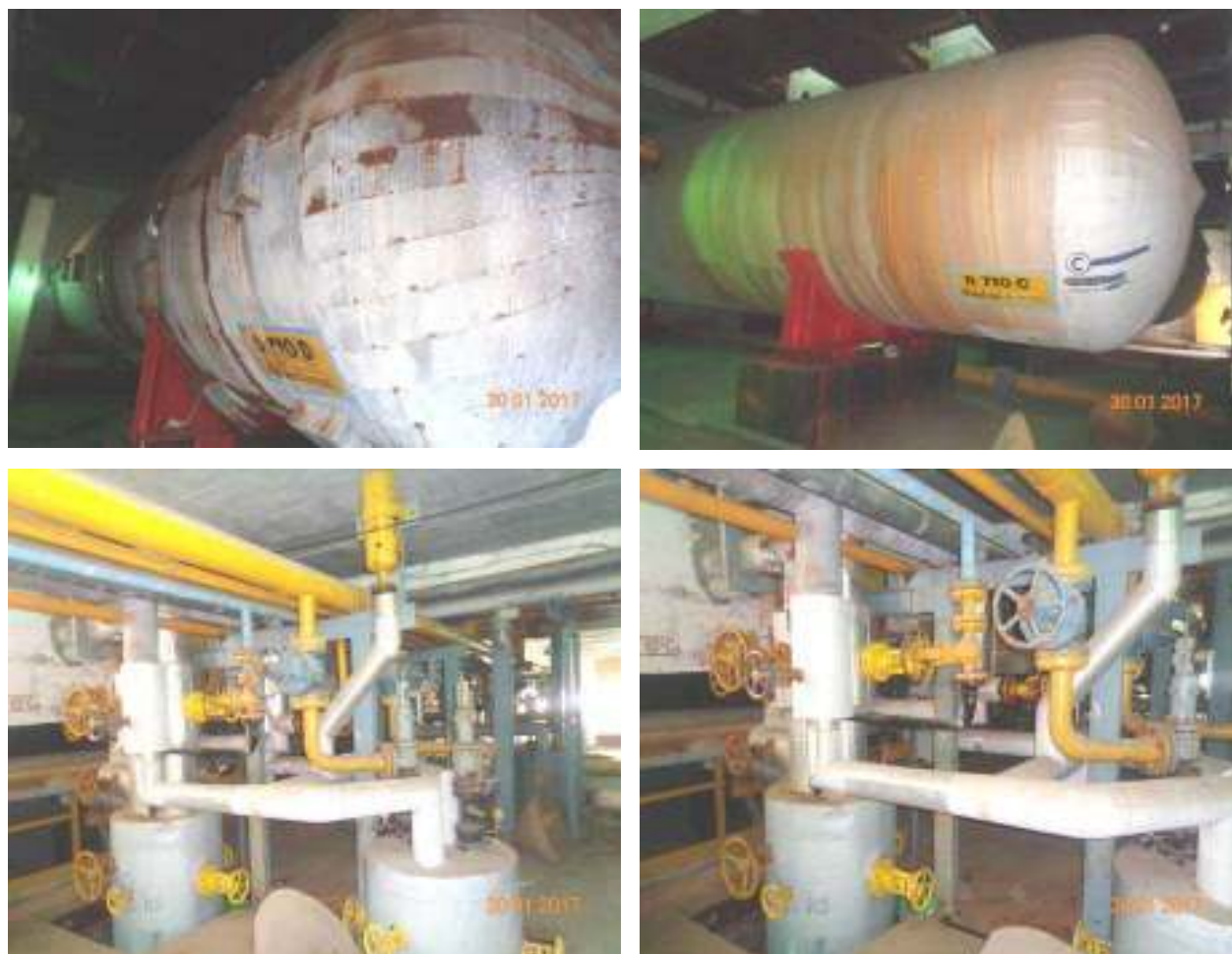
Fig 10.4 Chlorine storage tanks and Interlock system
