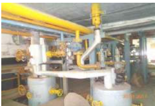
Fig 7.4 Chlorine storage tanks and Interlock system
